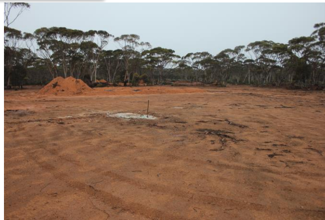
Cassini box-cut location cleared – 11 February 2020
