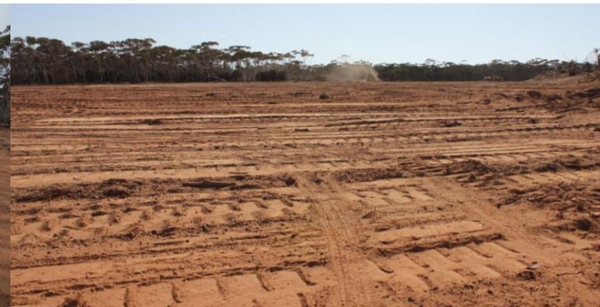
ROM pad clearing 1 March 2020
